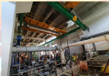
DOU Installation works at Preliminary Treatment Facilities in Progress 基本污水處理大樓的除臭系統及管道工程正在進行中
